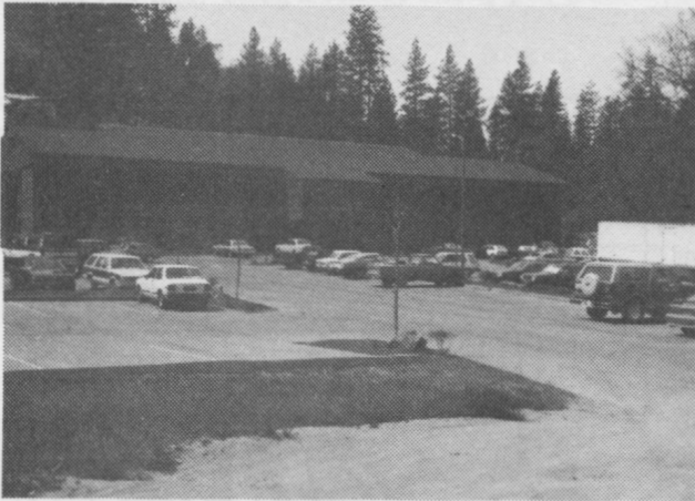
Sierra's current building is nestled amidst the pines of Oakhurst, California, at the southern gate of Yosemite National Park, the second largest national park in the United States.
